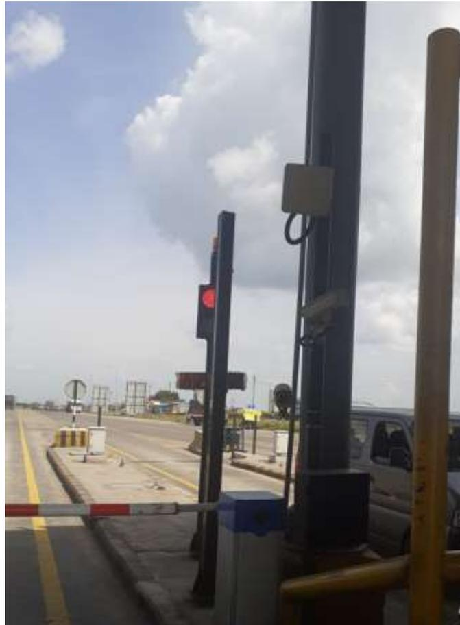
**Figure 9-2 RFID ETC Reader mounted on Pole**
