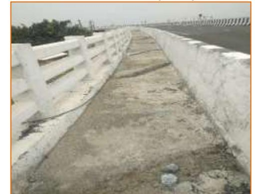
**Uneven Drain with footpath at A1
