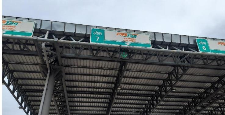
**Figure 9-9 Over Head Lane Signal (OHLS)**
