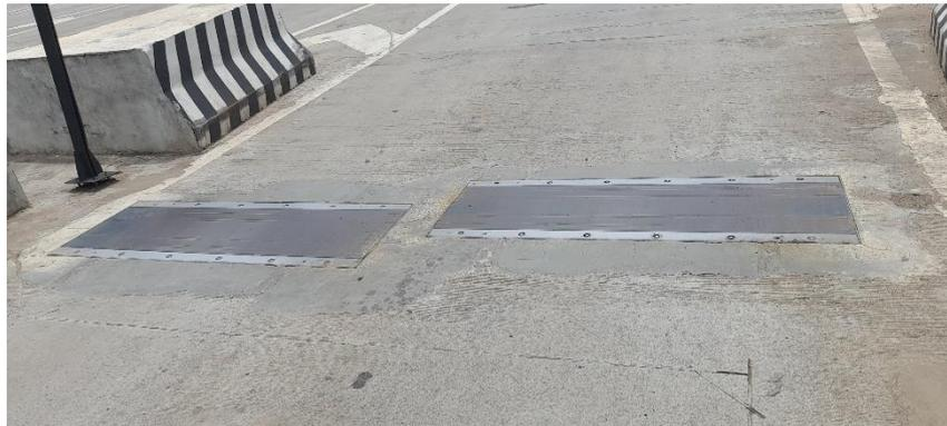
**Figure 9-11 Medium Speed Weigh in Motion (MSWIM)**
