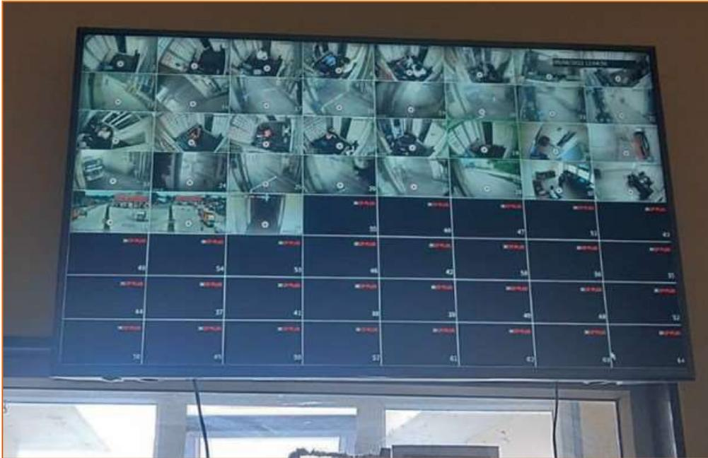
**Figure 9-5 55" LED screen for CCTV monitoring**
