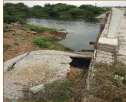
**Damaged CC Pitching of MNB at km. 456+533 (BHS) on Both end**
