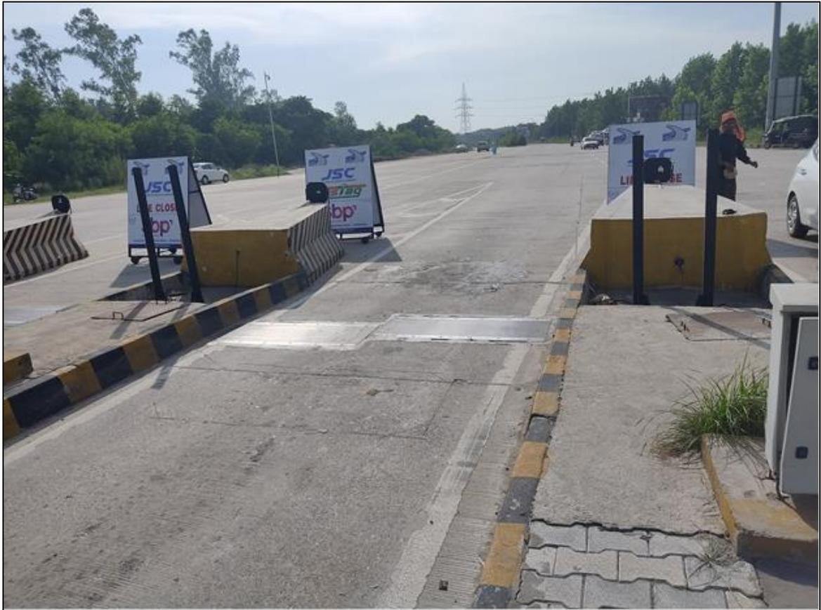
**Figure 9-12 Medium Speed Weigh in Motion (MSWIM)**
