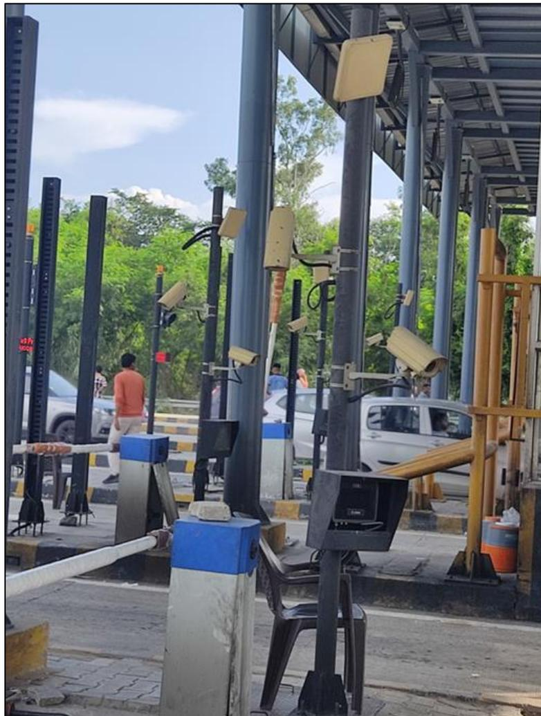
**Figure 9-3 RFID ETC Transceiver installed on pole**
