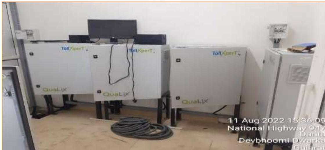
Figure 8-3 Lane Controllers for normal ETC lanes
