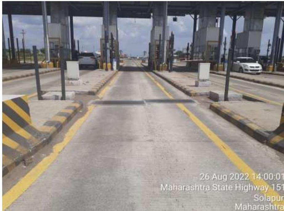
Figure 9-7 Medium Speed Weigh in Motion
