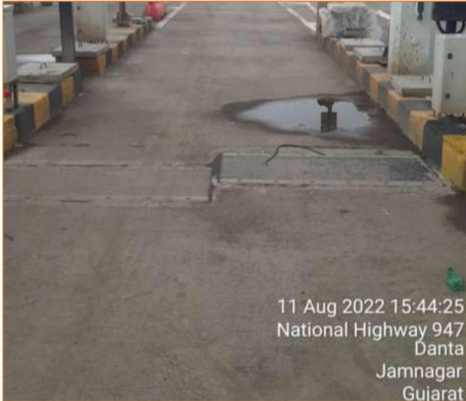
Figure 8-7 Medium Speed Weigh in Motion (MSWIM)
