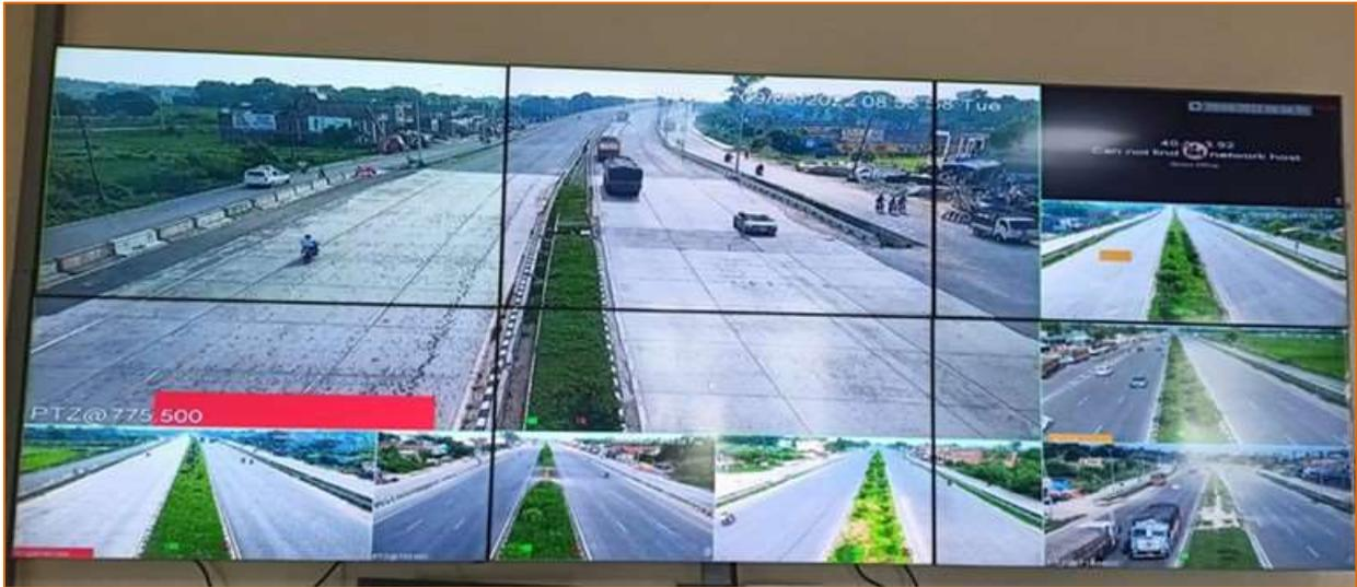
**Figure 9-10 Video wall in ATMS control centre**
