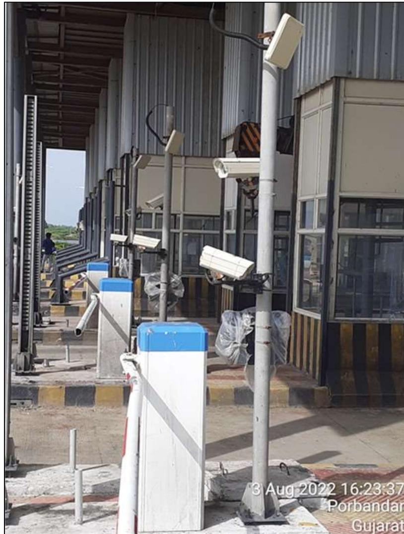
Figure 9-3 RFID ETC Reader mounted on Pole
