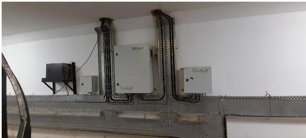
**Figure 9-3 Lane Controller and AVC installed in enclosures at Toll Booth**
