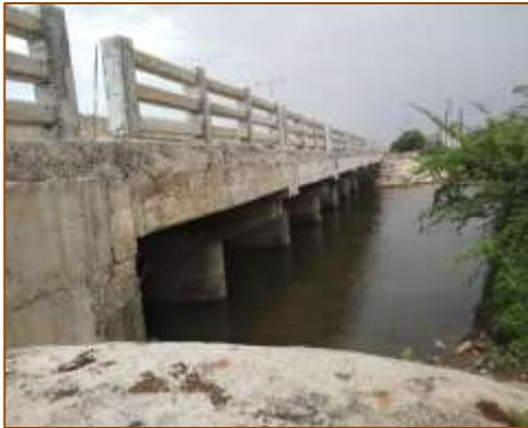
**Side View of Minor Bridge at km. 455+195 (LHS) - Missing railing**
