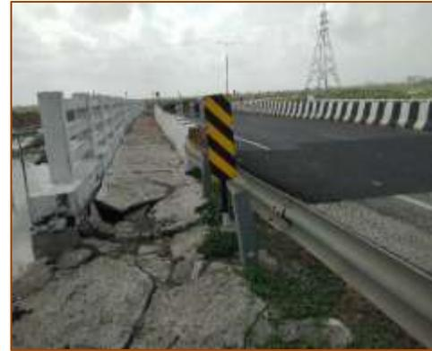
**Side View of Minor Bridge at km. 492+030 (RHS) - New - Footpath damaged**
