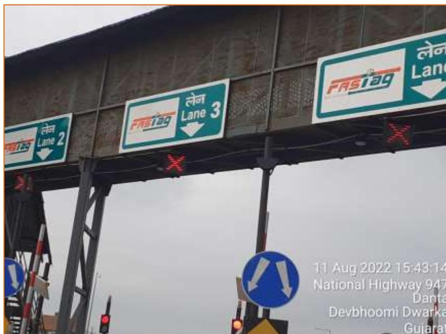
Figure 8-5 Over Head Lane Signal (OHLs)
