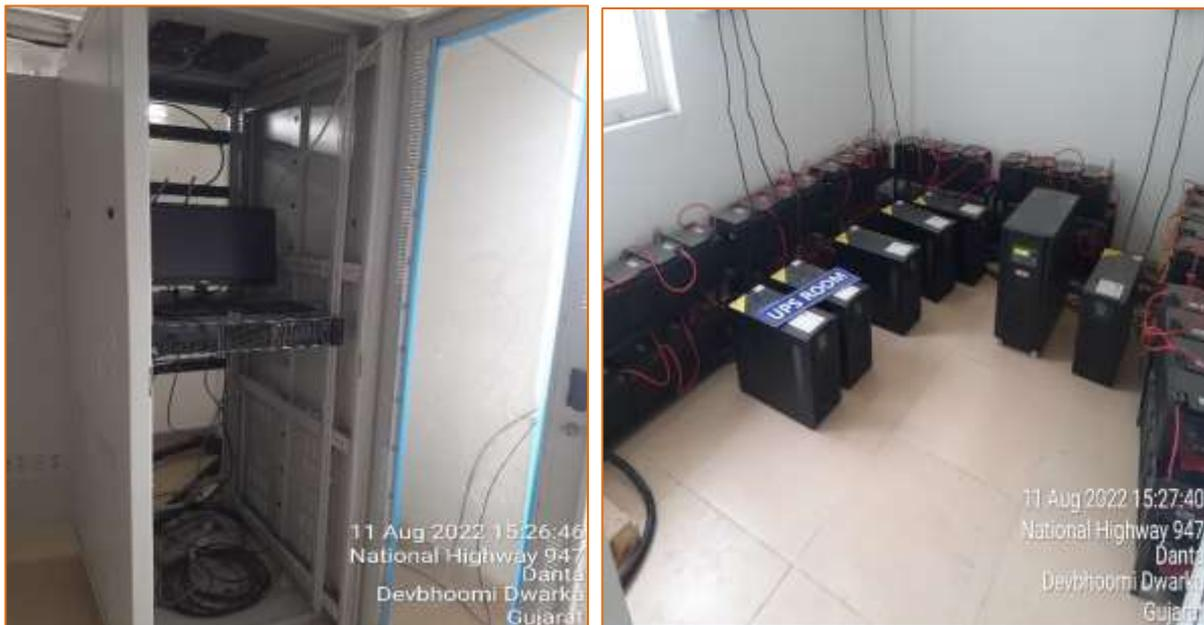
Figure 8-8 Control Room Equipment - Server & Switch rack/UPS Room
