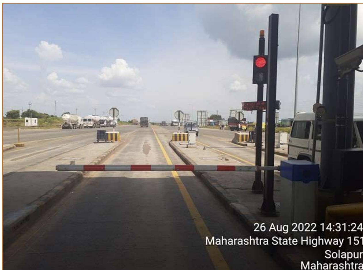
Figure 9-4 Automatic Lane Barrier
