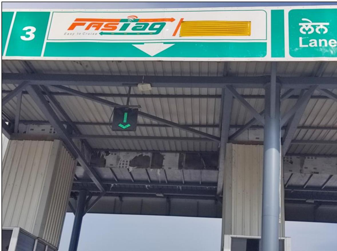
Figure 9-10 Over Head Lane Signal (OHLs)
