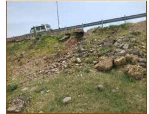
**Rain cuts developed at A2 side
