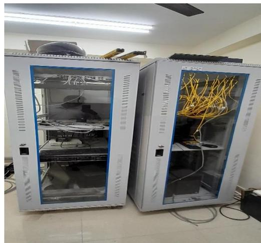
**Figure 9-12 Control Room Equipment - Server & Switch rack**
