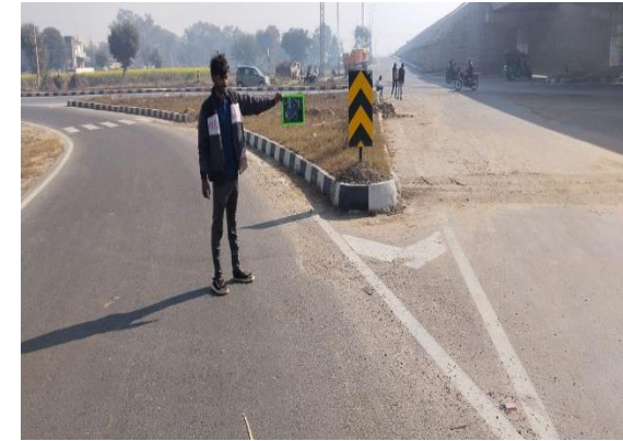
Fig 4.153: Junction at Ch 45+710 RHS
