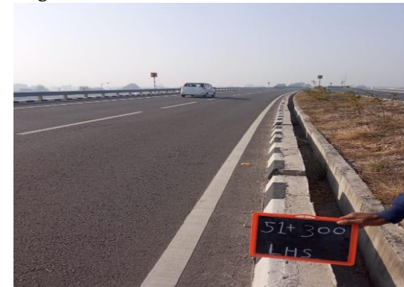
Fig 4.177: RCC Drain at Ch 51+300
