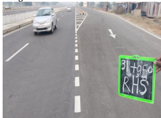
Fig 4.113: Service road at Ch 31+950 RHS Ateli- Narnaul
