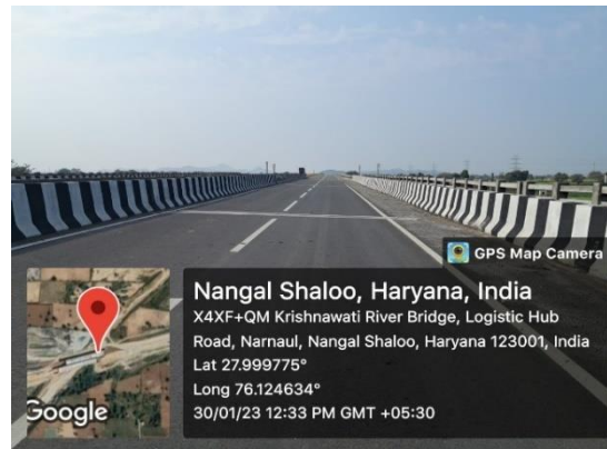
Fig 4.262: MJB at Ch. 2+130 LHS
