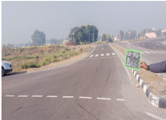
Fig 4.142: Junction at Ch 29+030 LHS
