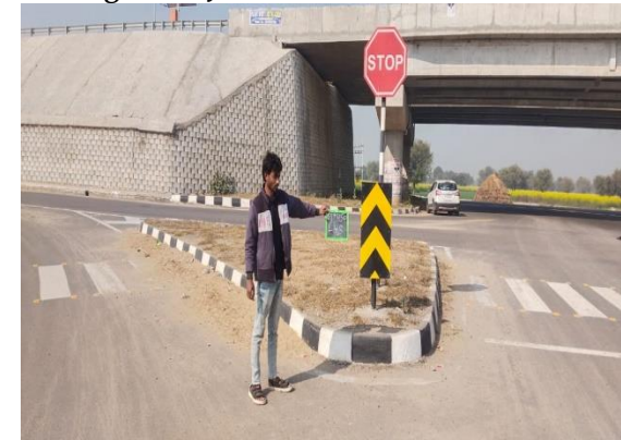
Fig 4.156: Junction at Ch 51+450 LHS
