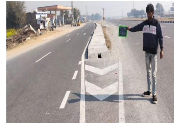
Fig 4.183: RCC Toe Drain at Ch 52+550 RHS
