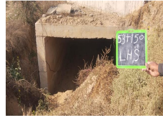
Fig 4.378: Box Culvert at Ch 53+150 LHS
