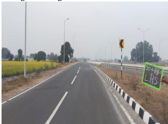
Fig 4.196: Sign Board at Ch 30+840 LHS
