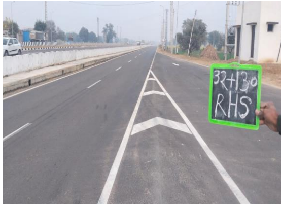
Fig 4.172: RCC Toe Drain at Ch 32+130 RHS
