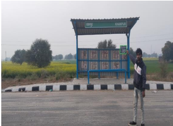
Fig 4.157: Busbay at 31+400 LHS
