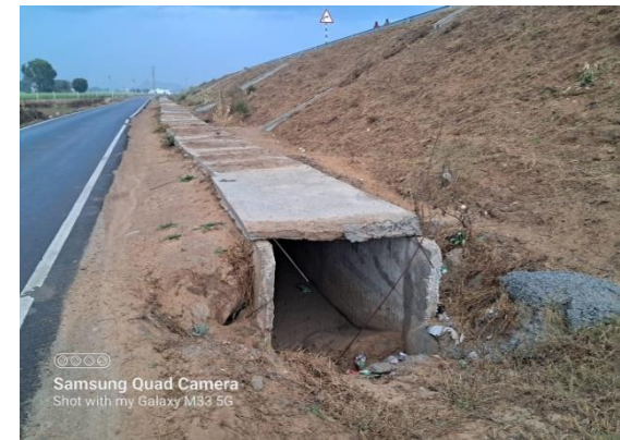
Fig 4.126: Service road at Ch 1+420 RHS
