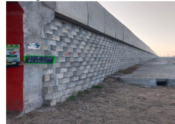
Fig 4.281: VUP at Ch.46+130
