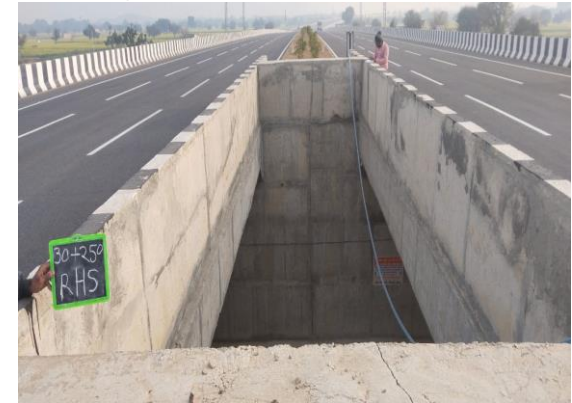
Fig 4.316: LVUP at Ch.30+250 RHS
