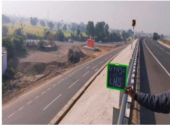
Fig 4.295: VUP at Ch 51+450 LHS
