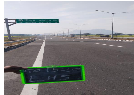
Fig 4.203: Sign Board at Ch 50+520 LHS
