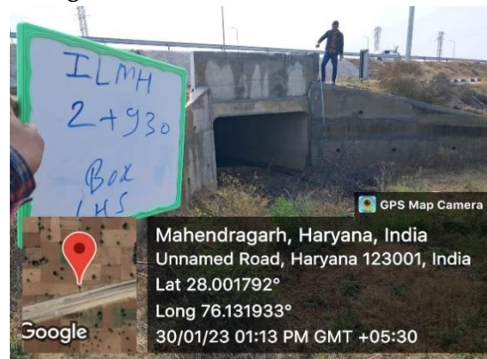
Fig 4.386: Box Culvert at Ch 2+930 LHS
