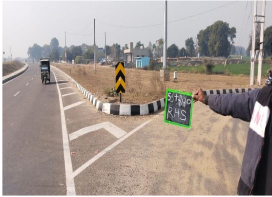
Fig 4.139: Junction at Ch 55+200 RHS
