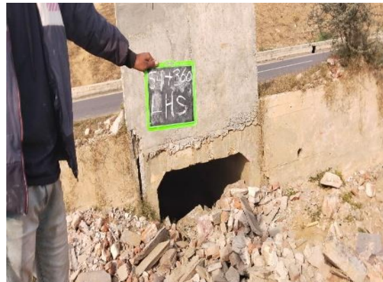
Fig 4.380: Box Culvert at Ch 54+360 LHS ILMH
