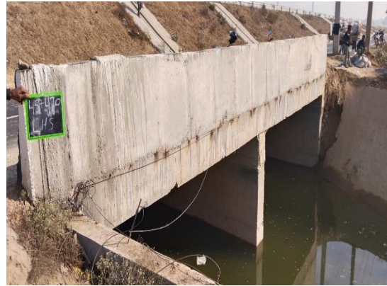
Fig 4.271: MNB at Ch. 45+470 LHS
