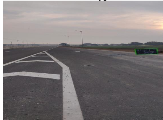
Fig 4.158: Busbay at 31+450 LHS
