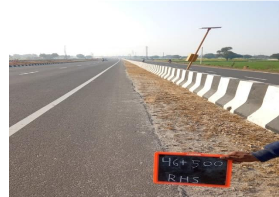
Fig 4.233: SOS Box at 46+500 RHS
