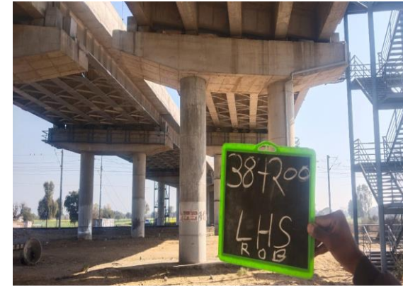
Fig 4.351: ROB at Ch 38+200 LHS
