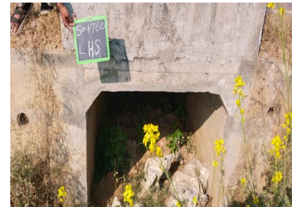
Fig 4.375: Box Culvert at Ch 50+760 LHS
