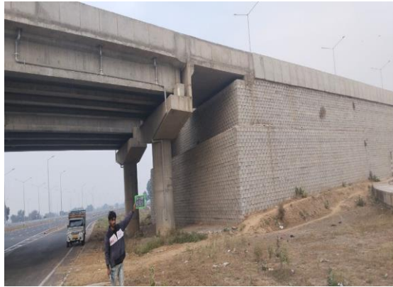
Fig 4.276: VUP at Ch 30+840 RHS
