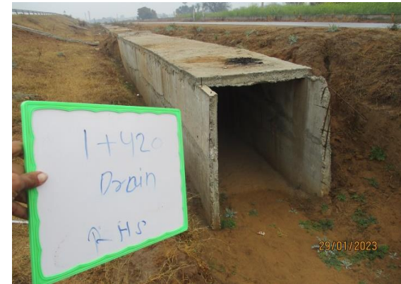
Fig 4.189: RCC Drain at Ch 1+420 RHS
