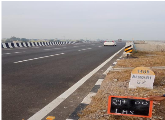
Fig 4.169: Drain at Ch 29+000
