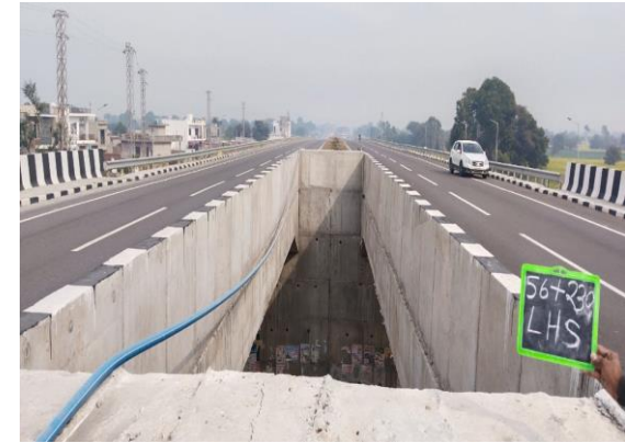
Fig 4.302: VUP at Ch. 56+230 LHS
