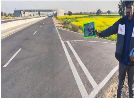
Fig 4.151: Junction at Ch 41+220 LHS
