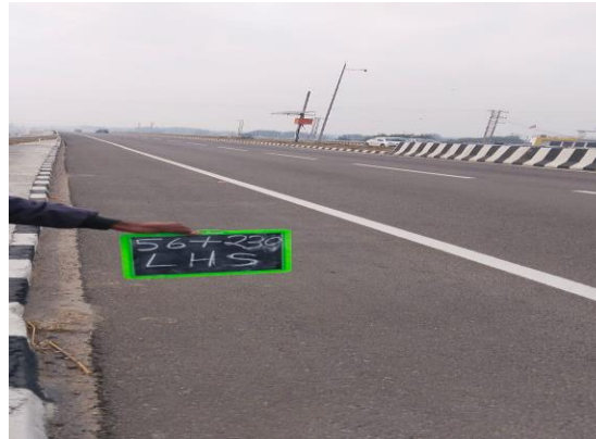
Fig 4.229: Camera with solar panel at Ch 56+230
