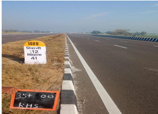
Fig 4.219: KM Stones at Ch 35+000
