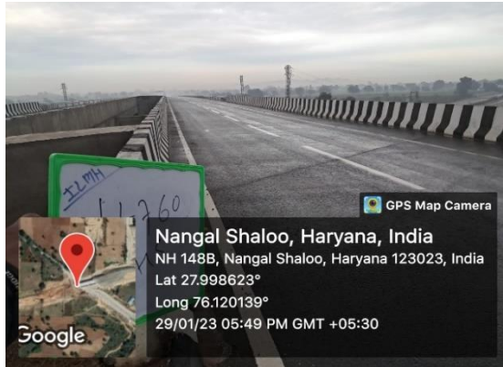
Fig 4.306: VUP at Ch 1+760 LHS
