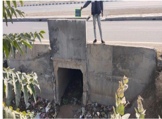
Fig 4.377: Box Culvert at Ch 52+930 RHS
