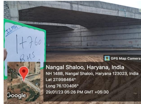
Fig 4.304: VUP at Ch 1+760 RHS
