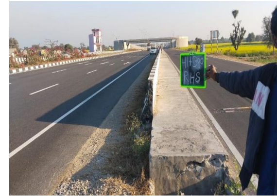
Fig 4.174: RCC Toe Drain at Ch 41+300 RHS
