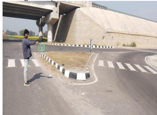
Fig 4.155: Junction at Ch 51+450 LHS
