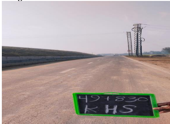
Fig 4.118: Service road at Ch 49+830 RHS
