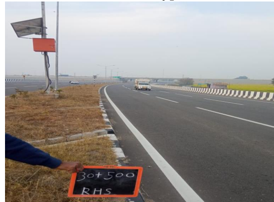
Fig 4.170: RCC Toe Drain at Ch 30+500
