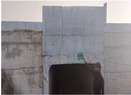
Fig 4.370: Box Culvert at Ch 46+470 RHS
