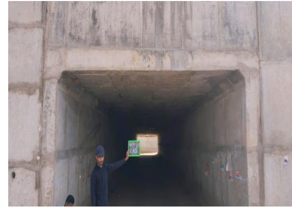
Fig 4.319: Subway at Ch. 46+580
