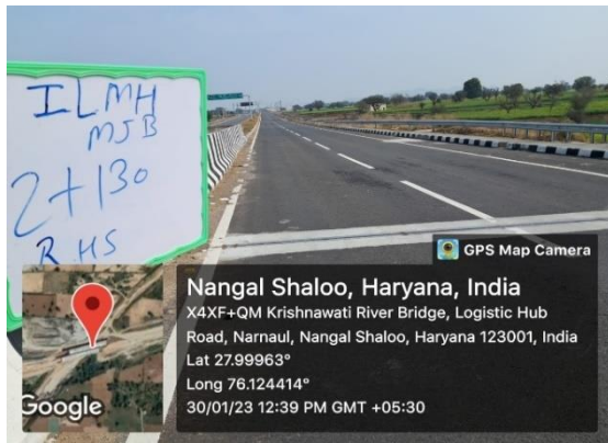
Fig 4.261: MJB at Ch. 2+130 RHS
