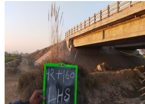
Fig 4.269: MNB at Ch. 42+160 LHS
