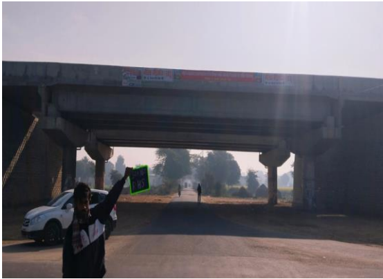
Fig 4.288: VUP at Ch.50+160 RHS
