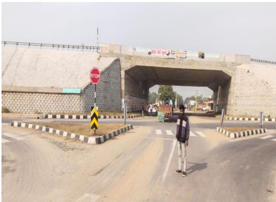
Fig 4.297: VUP at Ch. 54+050 LHS
