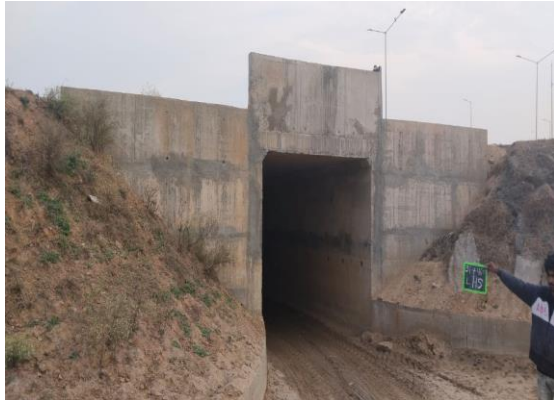
Fig 4.358: Box Culvert at Ch 31+460 LHS
