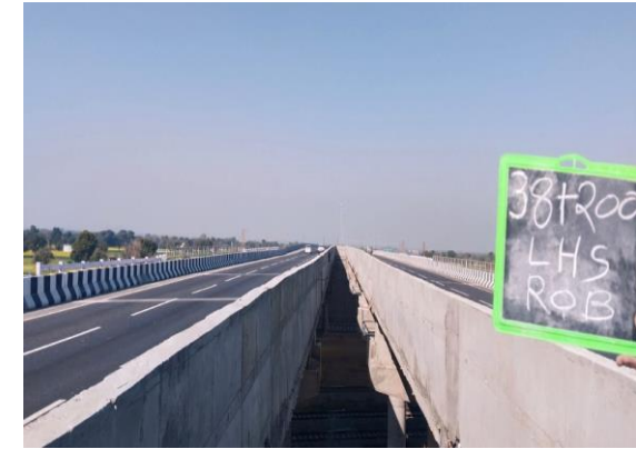
Fig 4.357: ROB at Ch 38+200 LHS
