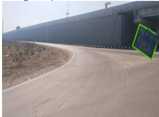
Fig 4.149: Junction at Ch 36+160 RHS
