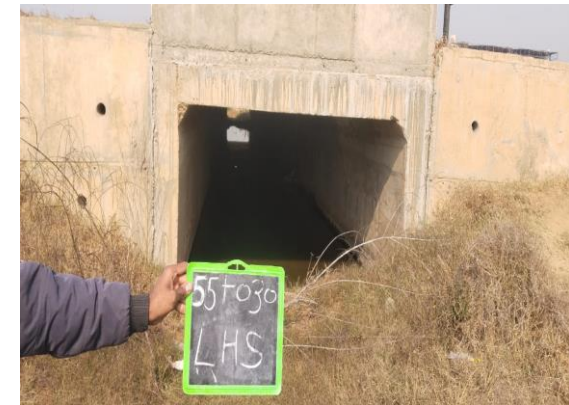
Fig 4.381: Box Culvert at Ch 55+030 LHS
