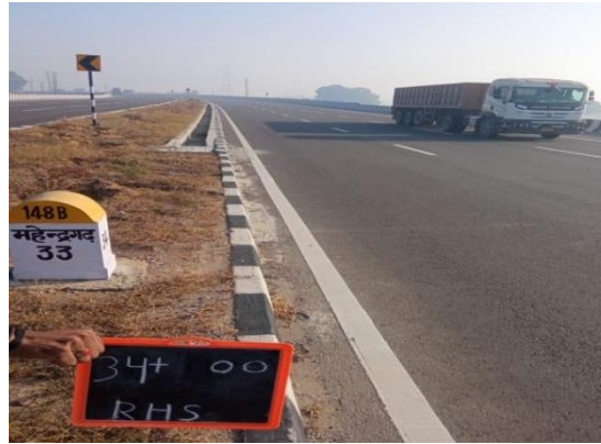
Fig 4.199: Sign Board at Ch 34+000 RHS
