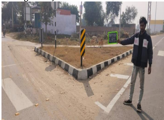
Fig 4.136: Junction at Ch 54+050 LHS
