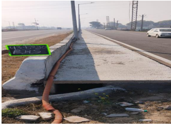
Fig 4.178: Drain at Ch 43+8730 RHS
