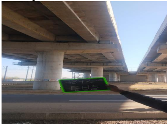
Fig 4.353: ROB at Ch 38+200 RHS
