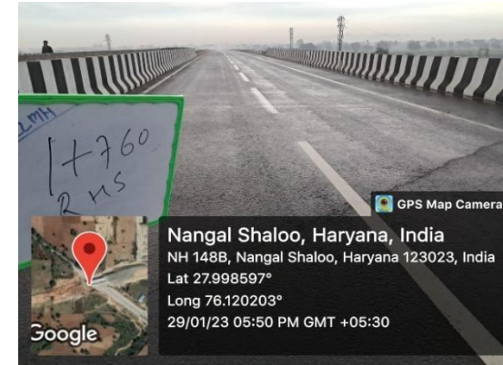
Fig 4.307: VUP at Ch 1+760 RHS
