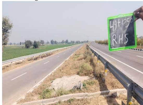
Fig 4.176: RCC Drain at Ch 49+050 RHS Ateli- Narnaul
