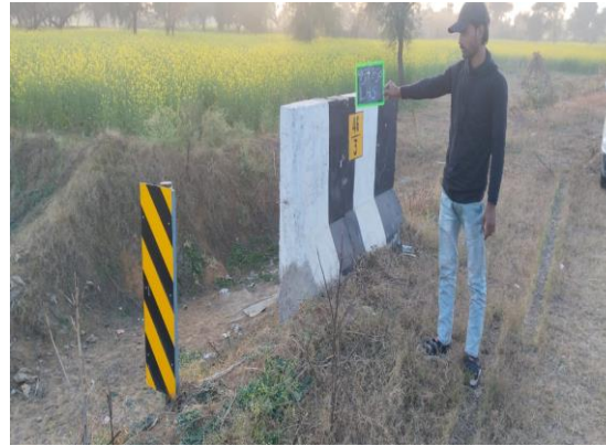
Fig 4.365: Box Culvert at Ch 45+850 LHS
