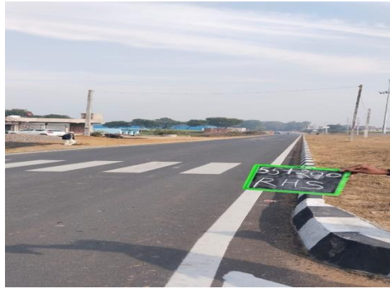
Fig 4.122: Service road at Ch 55+200 RHS
