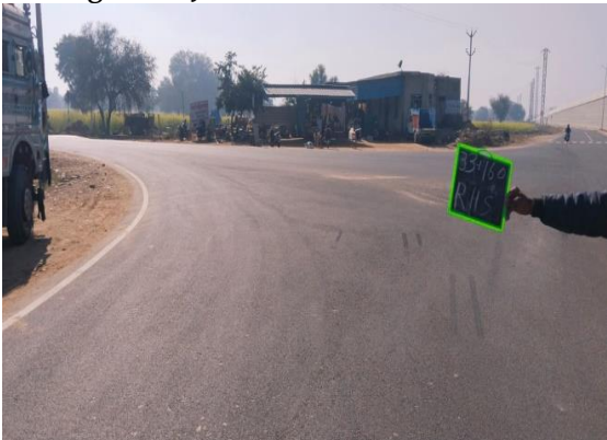
Fig 4.148: Junction at Ch 33+160 RHS
