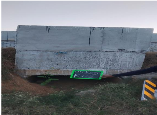
Fig 4.364: Box Culvert at Ch 45+850 RHS
