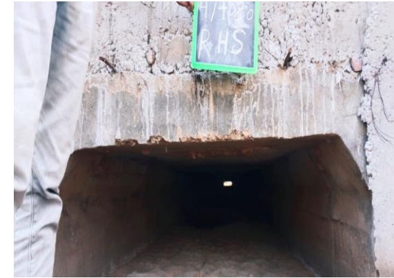
Fig 4.366: Box Culvert at Ch 47+080 RHS
