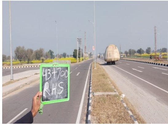
Fig 4.116: Service road at Ch 43+700 RHS
