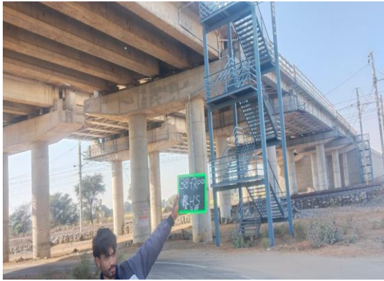
Fig 4.349: ROB at Ch 38+200 RHS
