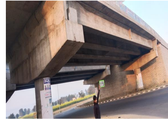
Fig 4.278: VUP at Ch. 45+140 LHS
