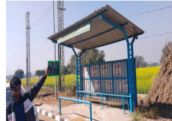
Fig 4.159: Busbay at 32+900 LHS
