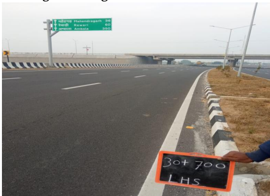
Fig 4.195: Sign Board at Ch 30+700 LHS
