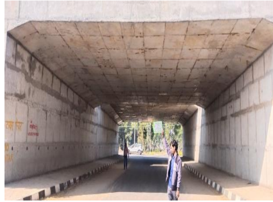
Fig 4.309: LVUP at Ch. 34+480 RHS Narnaul Bypass
