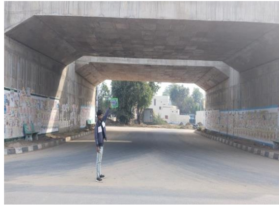
Fig 4.301: VUP at Ch. 56+230 RHS ILMH
