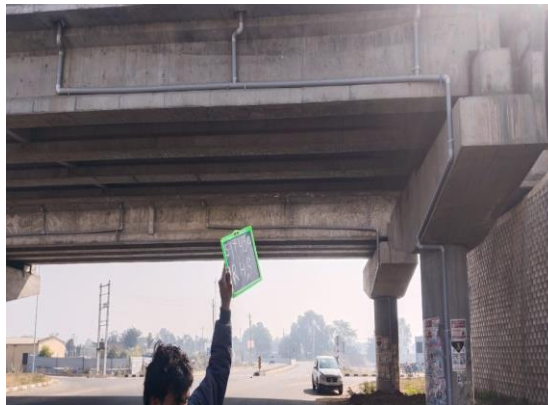
Fig 4.292: VUP at Ch 51+450 RHS
