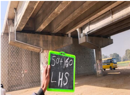
Fig 4.291: VUP at Ch.50+160 LHS
