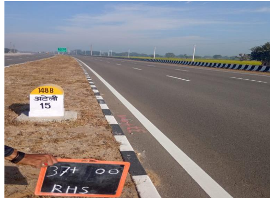
Fig 4.220: KM Stones at Ch 37+000
