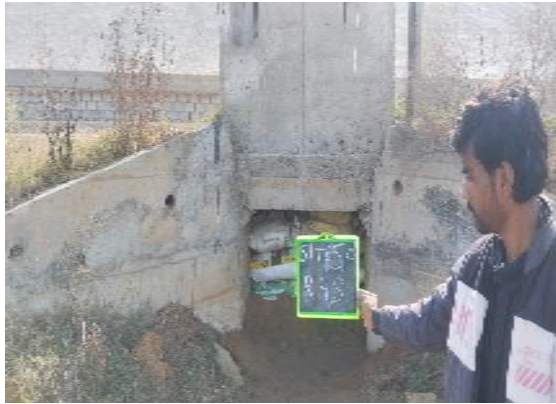
Fig 4.376: Box Culvert at Ch 51+650 RHS
