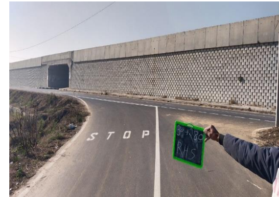
Fig 4.144: Junction at Ch 30+280 RHS
