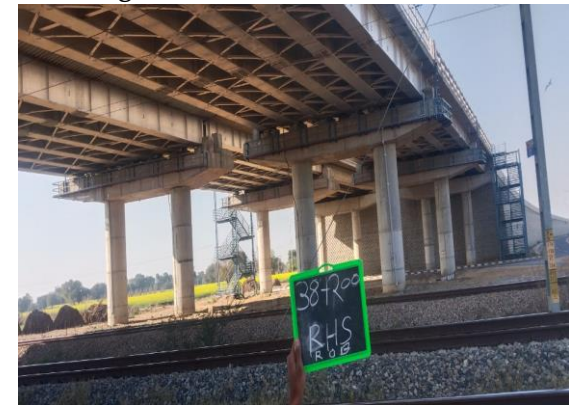
Fig 4.354: ROB at Ch 38+200 RHS
