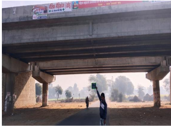
Fig 4.289: VUP at Ch.50+160 RHS
