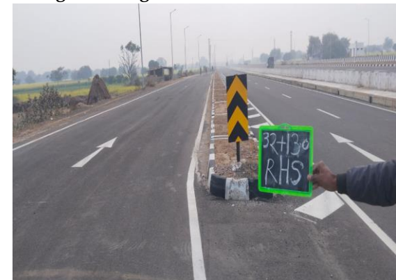
Fig 4.197: Sign Board at Ch 32+130 RHS
