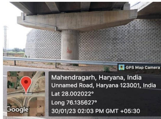
Fig 4.347: Flyover at Ch. 3+300
