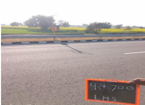
Fig 4.207: MBCB at Ch 42+700 LHS
