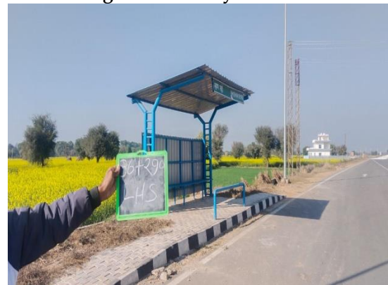
Fig 4.161: Busbay at 36+290 LHS
