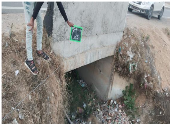
Fig 4.373: Box Culvert at Ch 48+000LHS
