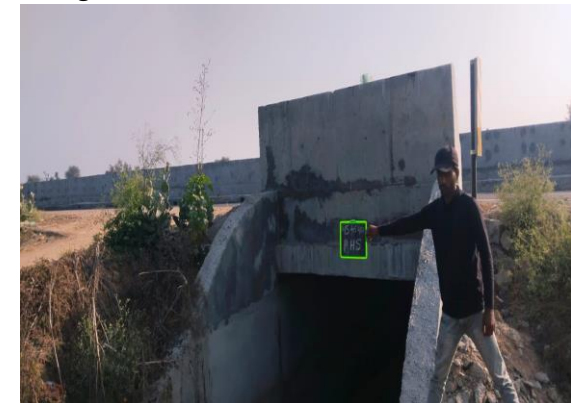
Fig 4.363: Box Culvert at Ch 45+640 RHS
