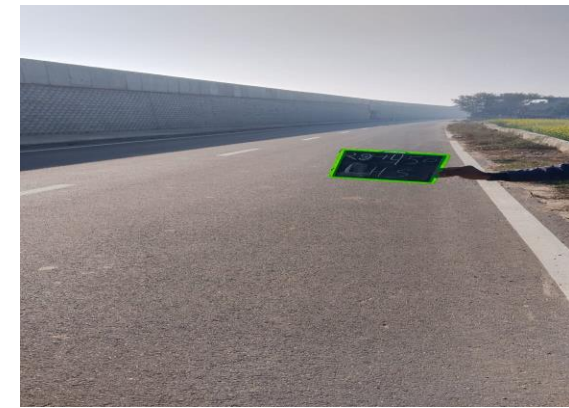
Fig 4.111: Service road at Ch 29+450 RHS
