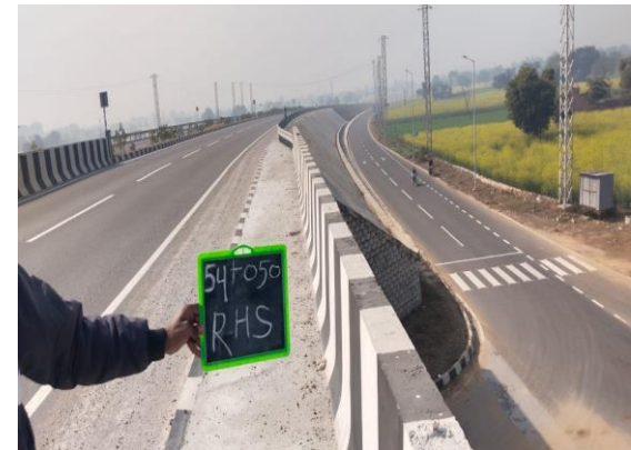
Fig 4.299: VUP at Ch. 54+050 RHS
