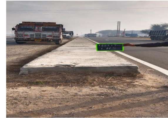
Fig 4.180: RCC Drain at Ch 48+130 LHS
