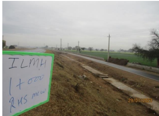
Fig 4.188: RCC Toe Drain at Ch 1+000 ILMH
