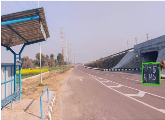
Fig 4.163: Busbay at 47+150 RHS
