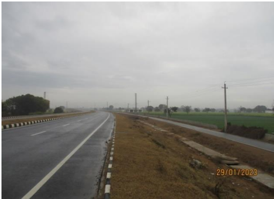
Fig 4.187: Drain at C 1+000 RHS
