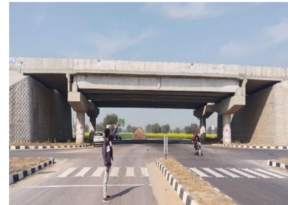
Fig 4.293: VUP at Ch 51+450 LHS
