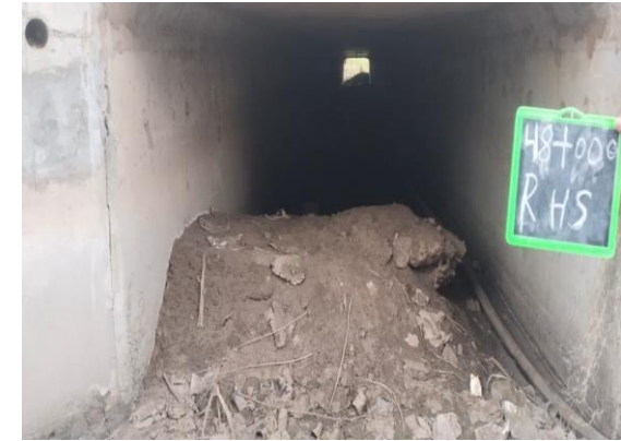
Fig 4.372: Box Culvert at Ch 48+000 RHS
