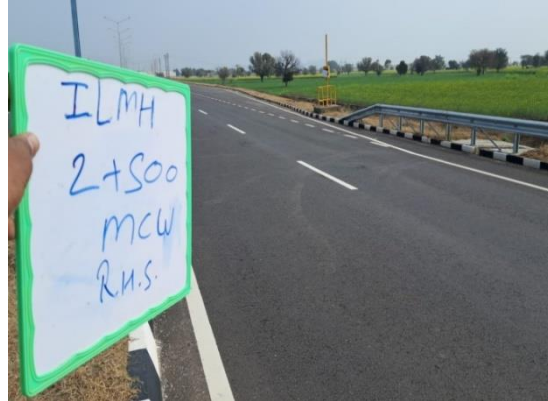
Fig 4.238: SOS Box at 2+500 RHS
