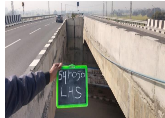
Fig 4.296 VUP at Ch. 54+050 LHS
