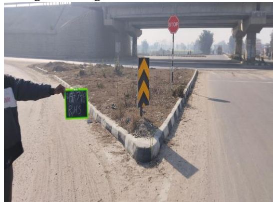
Fig 4.202: Sign Board at Ch 45+740 RHS
