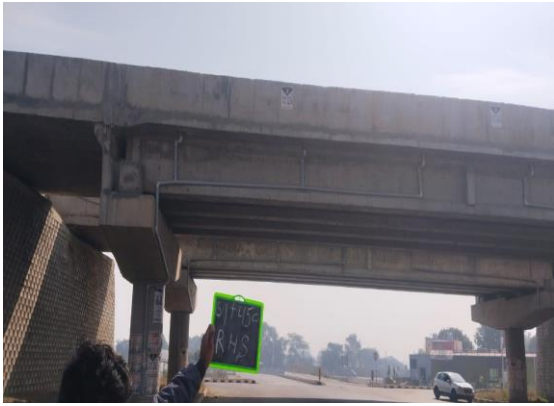
Fig 4.282: VUP at Ch. 51+450 RHS
