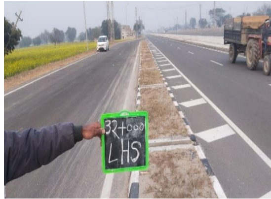
Fig 4.173: Drain at Ch 32+000
