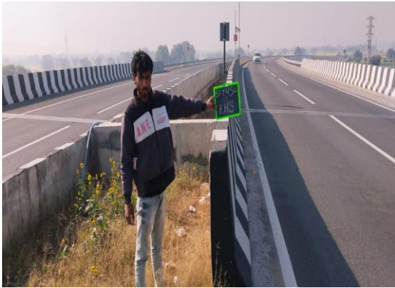
Fig 4.294: VUP at Ch 51+450 RHS
