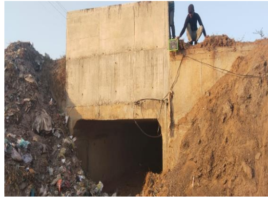
Fig 4.371: Box Culvert at Ch 46+470 LHS
