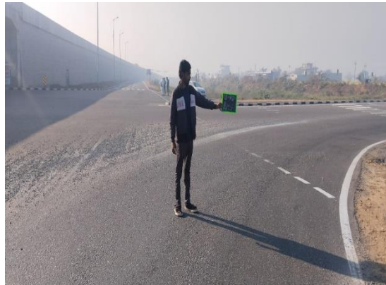
Fig 4.143: Junction at Ch 29+030 LHS
