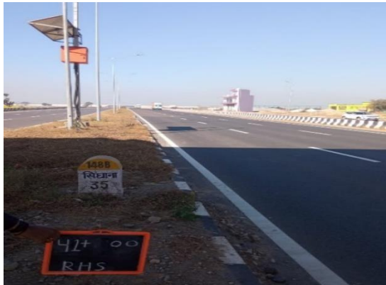
Fig 4.217: Lighting at Ch.42+000
