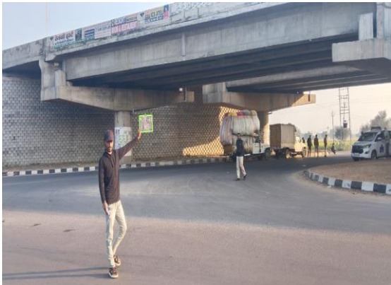
Fig 4.285: VUP at Ch. 47+540 RHS
