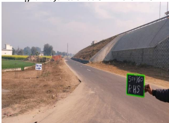
Fig 4.130: Junction at Ch 50+160 RHS
