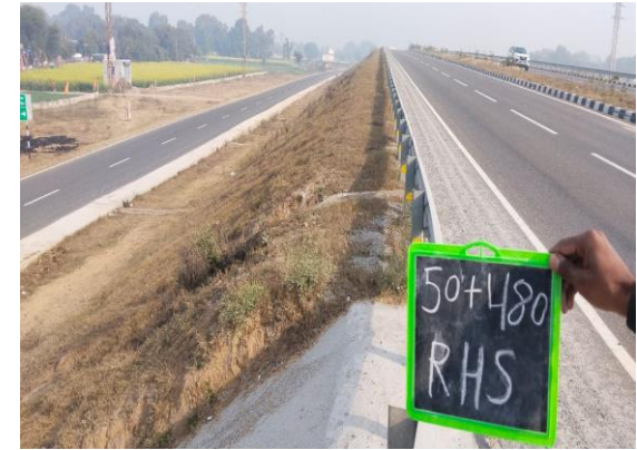
Fig 4.330: PUP at Ch.50+480 RHS
