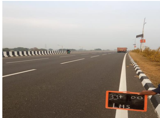
Fig 4.223: Camera with solar panel at Ch 33+000
