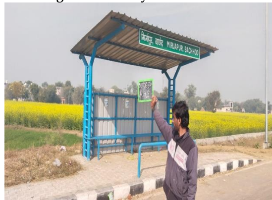
Fig 4.167: Busbay at 53+650 RHS
