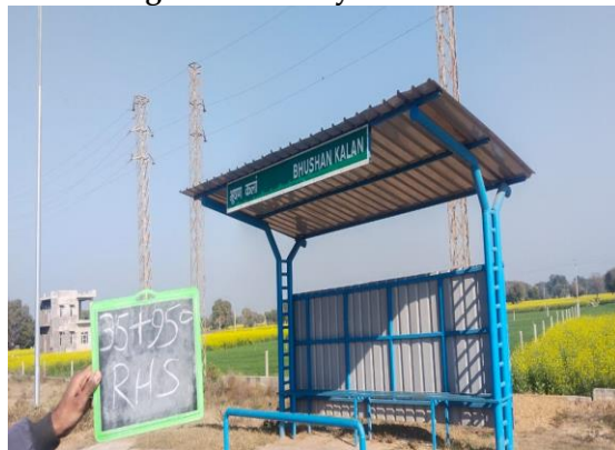
Fig 4.160: Busbay at 35+950 RHS
