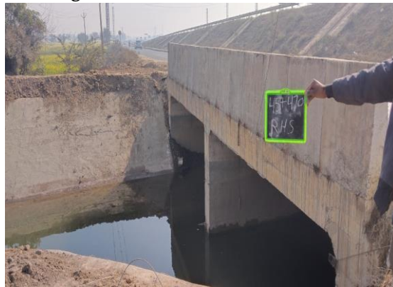
Fig 4.273: MNB at Ch. 45+470 RHS
