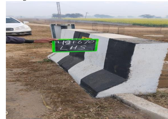
Fig 4.369: Box Culvert at Ch 49+670 LHS
