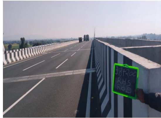
Fig 4.356: ROB at Ch 38+200 RHS
