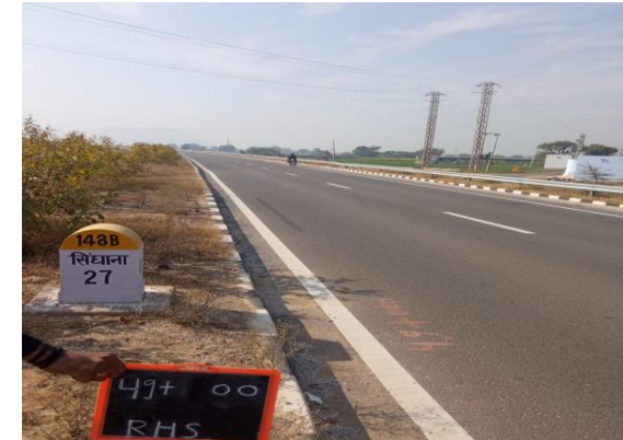
Fig 4.221: KM Stones at Ch 49+000
