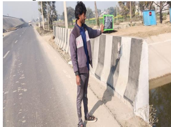
Fig 4.274: MNB at Ch. 45+470 RHS
