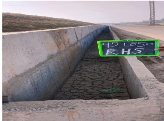
Fig 4.185: RCC Drain at Ch 49+850 RHS ILMH
