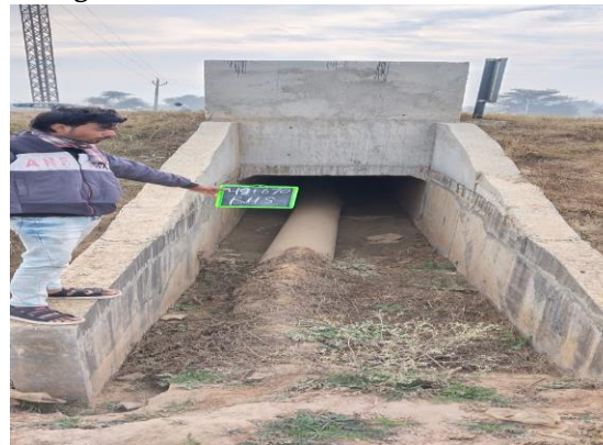
Fig 4.368: Box Culvert at Ch 49+670 RHS Ateli - Narnaul
