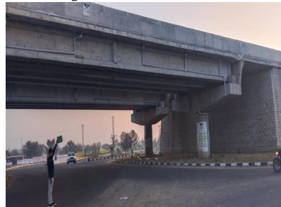
Fig 4.280: VUP at Ch. 45+140
