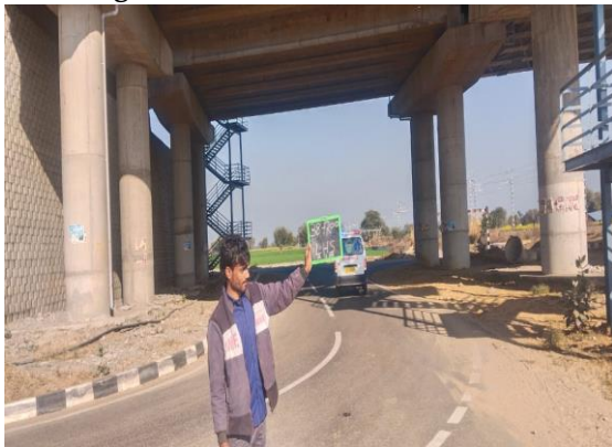
Fig 4.352: ROB at Ch 38+200 LHS
