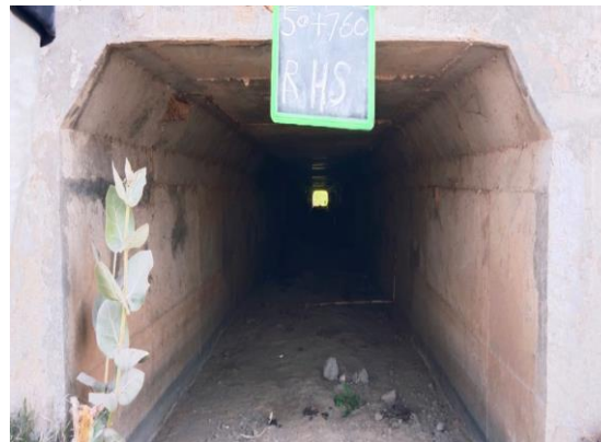
Fig 4.374: Box Culvert at Ch 50+760 RHS
