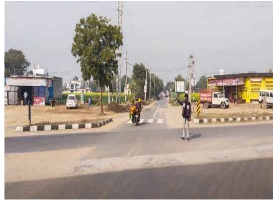
Fig 4.134: Junction at Ch 54+050 RHS
