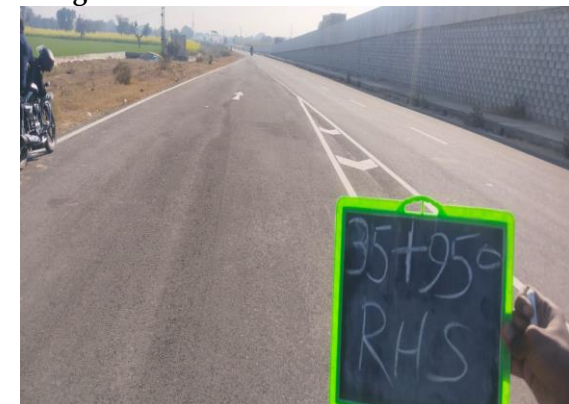
Fig 4.114: Service road at Ch 35+950 RHS
