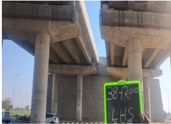
Fig 4.355: ROB at Ch 38+200 LHS
