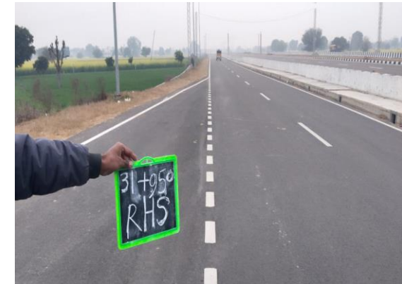
Fig 4.171: RCC Drain at Ch 31+950 RHS
