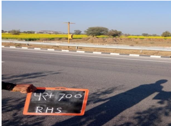
Fig 4.208: MBCB at Ch 42+700
