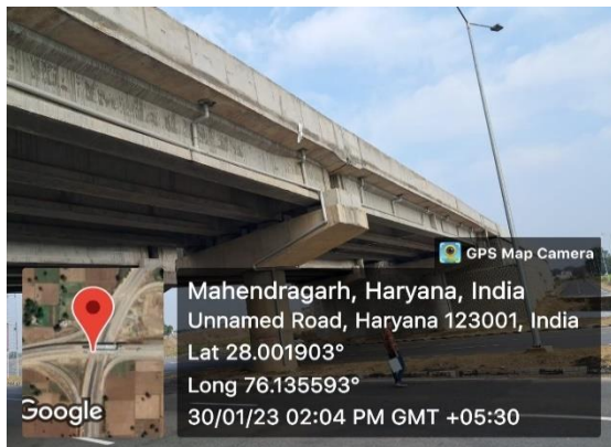
Fig 4.346: Flyover at Ch. 3+300
