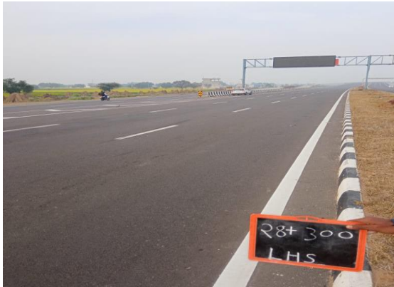
Fig 4.192: Sign Board at 28+300 LHS
