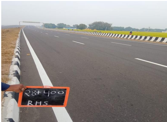
Fig 4.204: RCC crash barriers at Ch 28+400 RHS
