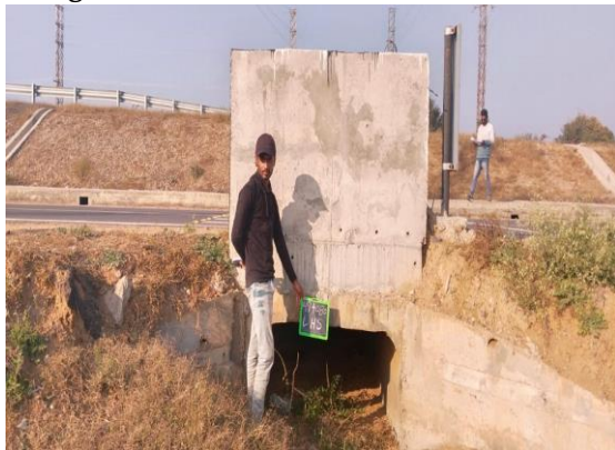
Fig 4.367: Box Culvert at Ch 47+080 LHS
