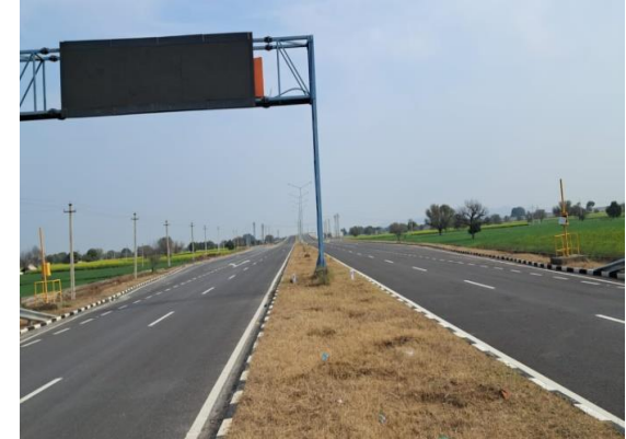
Fig 4.239: SOS Box at 2+400BHS
