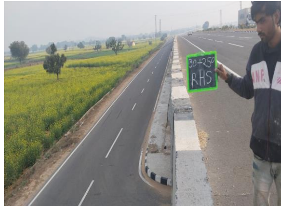
Fig 4.315: LVUP at Ch.30+250 RHS
