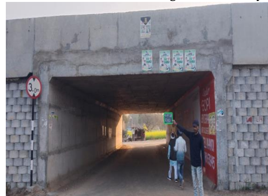
Fig 4.321: Subway at Ch. 32+207
