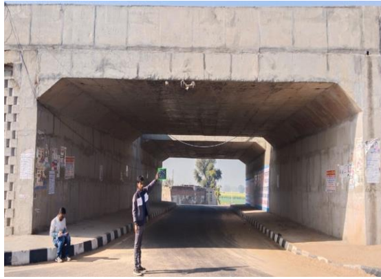
Fig 4.308: LVUP at Ch. 30+250 RHS Narnaul Bypass
