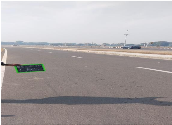
Fig 4.184: RCC Toe Drain at Ch 55+030 LHS
