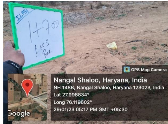
Fig 4.383: Box Culvert at Ch 1+700 LHS
