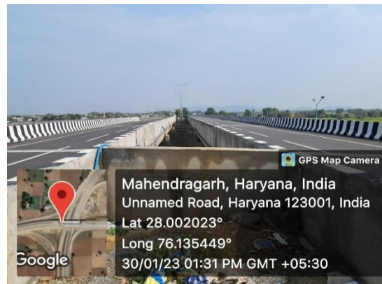
Fig 4.344: Flyover at Ch. 3+300
