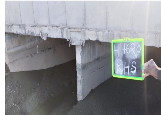
Fig 4.266: MNB at Ch. 41+620 RHS
