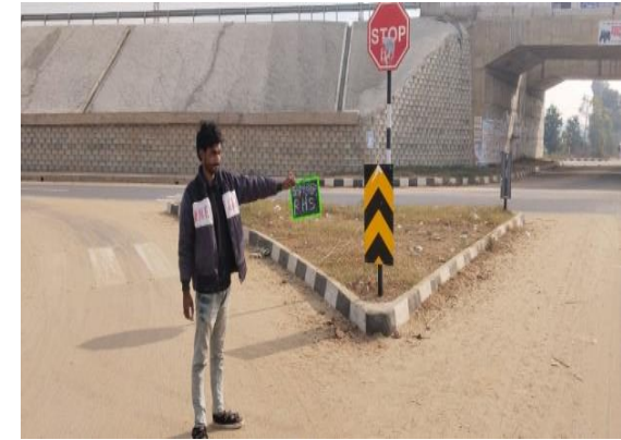
Fig 4.135: Junction at Ch 54+050 RHS
