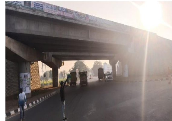
Fig 4.287: VUP at Ch. 47+540 LHS
