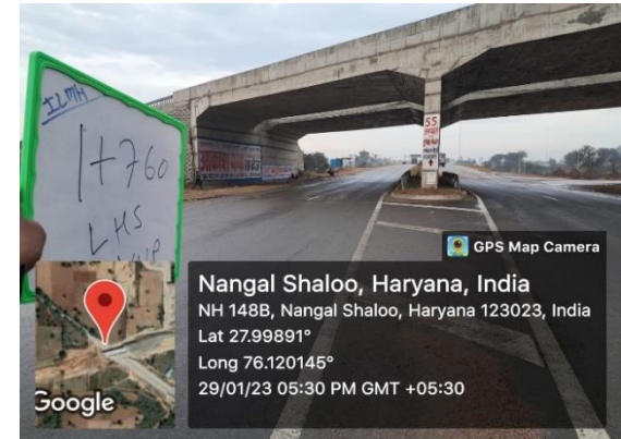
Fig 4.305: VUP at Ch 1+760 LHS
