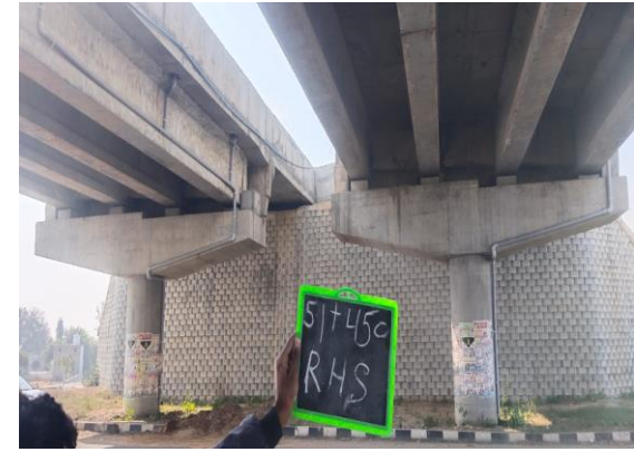
Fig 4.284: VUP at Ch. 51+450 RHS
