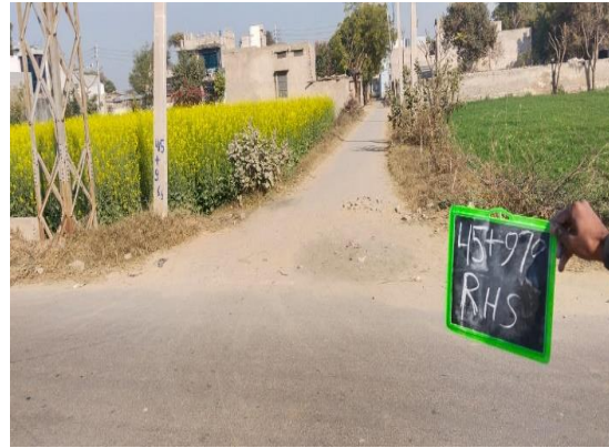
Fig 4.152: Junction at Ch 45+970 RHS
