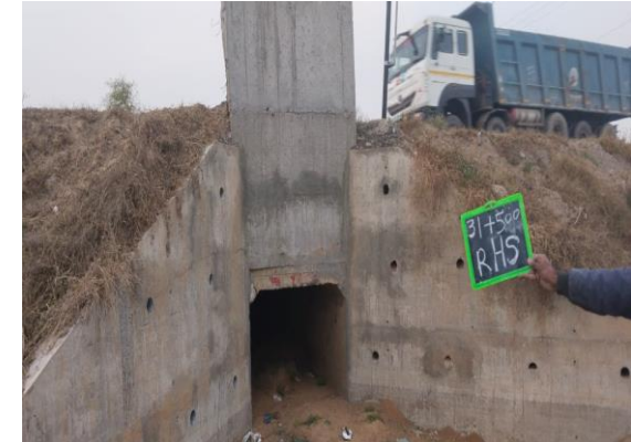
Fig 4.360: Box Culvert at Ch 31+500 RHS
