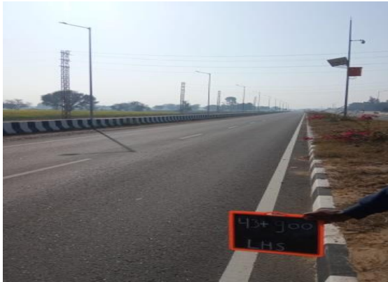
Fig 4.228: Camera with solar panel at Ch 44+900
