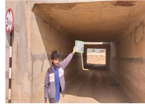
Fig 4.310: LVUP at Ch. 46+580 LHS Narnaul Bypass
