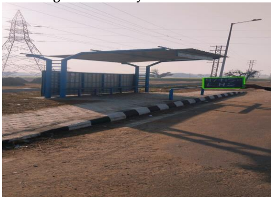
Fig 4.166: Busbay at 47+150 LHS
