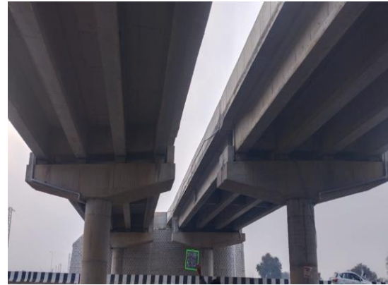
Fig 4.277: VUP at Ch. 30+840
