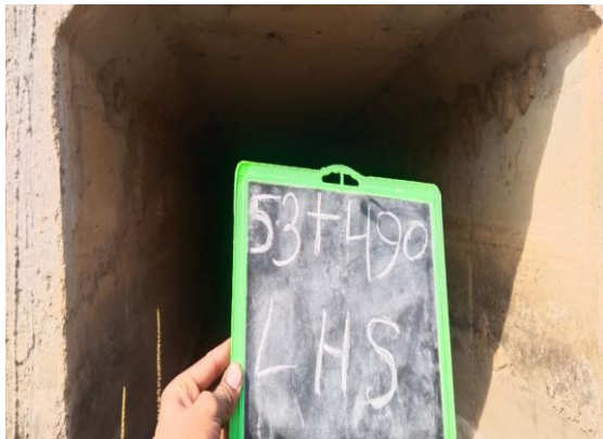
Fig 4.379: Box Culvert at Ch 53+490 LHS
