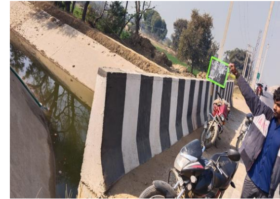
Fig 4.272: MNB at Ch. 45+470 LHS
