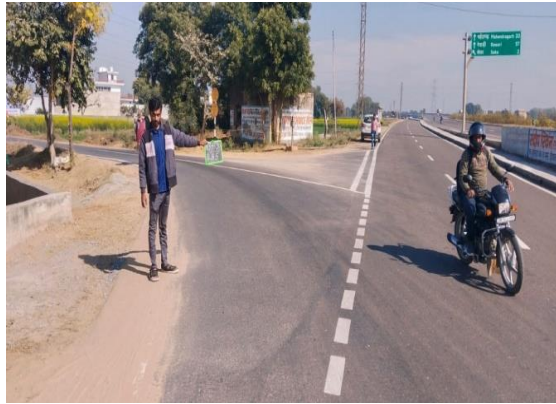
Fig 4.198: Sign Board at Ch 33+630 LHS
