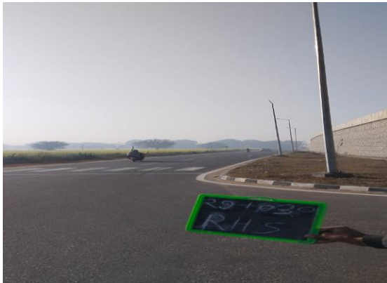
Fig 4.213: Lighting at Ch. 29+630 RHS
