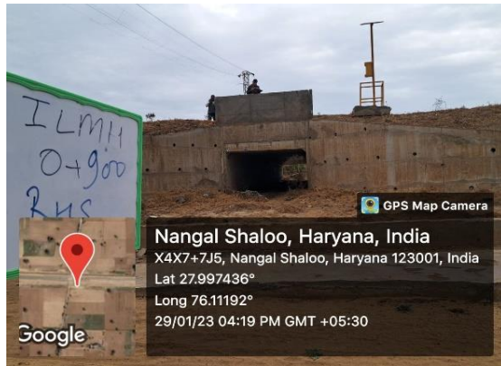
Fig 4.382: Box Culvert at Ch 0+900 RHS
