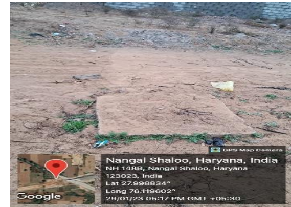
Fig 4.384: Box Culvert at Ch 1+700 LHS
