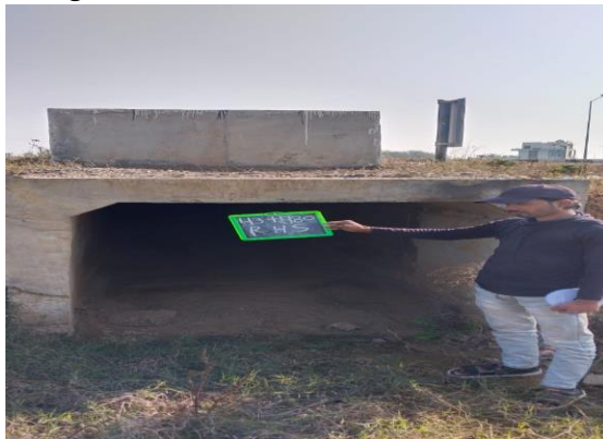
Fig 4.361: Box Culvert at Ch 43+480 RHS
