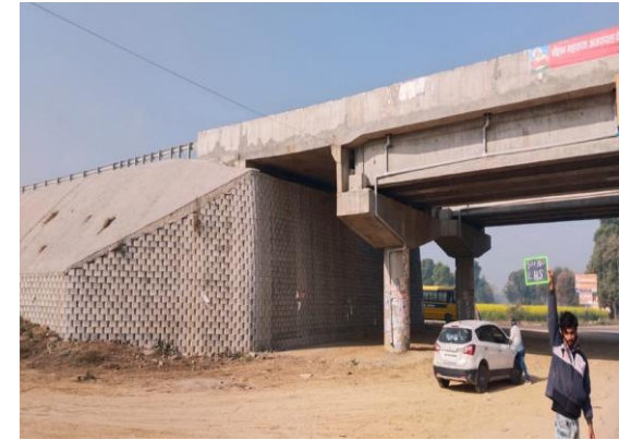
Fig 4.290: VUP at Ch.50+160 LHS
