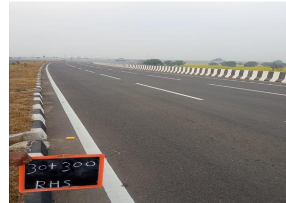
Fig 4.206: RCC crash barriers at Ch 30+300 RHS
