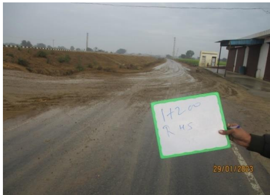
Fig 4.124: Service road at Ch 1+200 RHS
