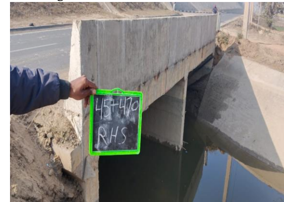
Fig 4.275: MNB at Ch. 45+470 RHS
