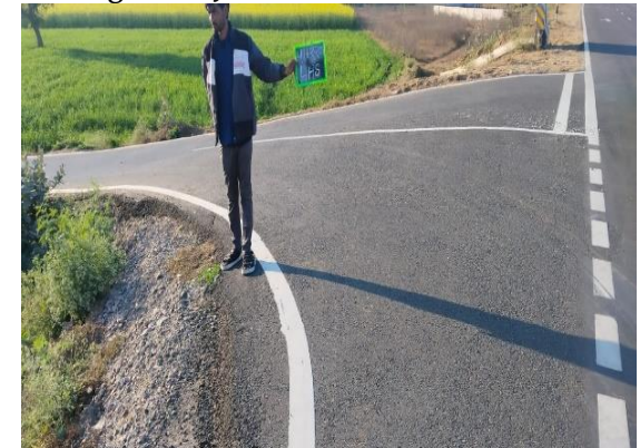
Fig 4.150: Junction at Ch 41+220 LHS
