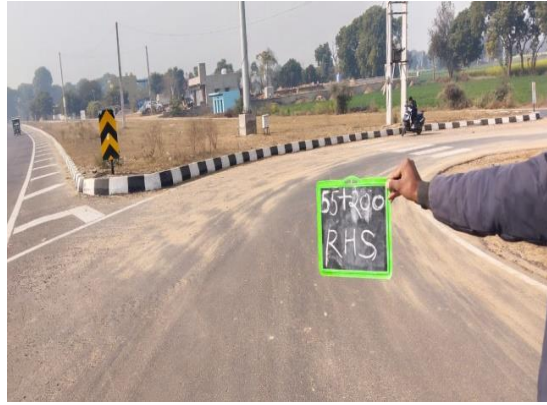
Fig 4.140: Junction at Ch 55+200 RHS NARNAUL BYPASS
