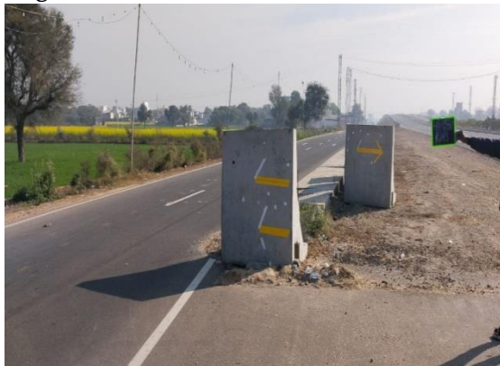
Fig 4.175: RCC Toe Drain at Ch 46+600 RHS
