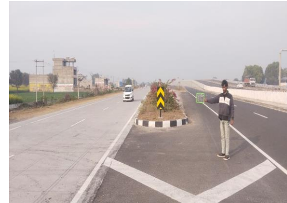
Fig 4.194: Sign Board at Ch 28+500 LHS
