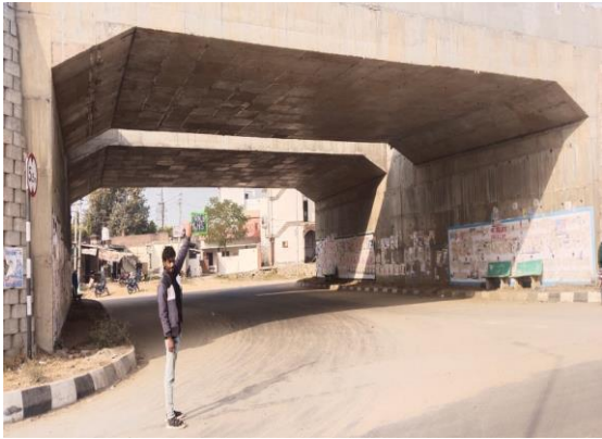
Fig 4.300: VUP at Ch. 56+230 LHS
