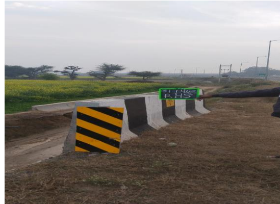
Fig 4.359: Box Culvert at Ch 31+460 RHS
