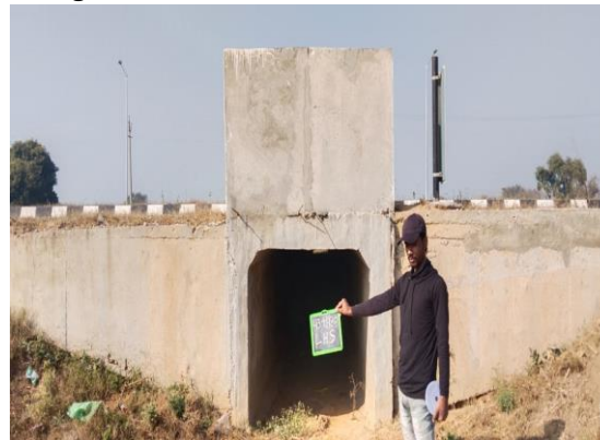
Fig 4.362: Box Culvert at Ch 43+480 LHS
