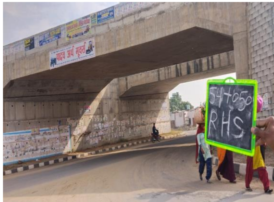
Fig 4.298: VUP at Ch. 54+050 RHS
