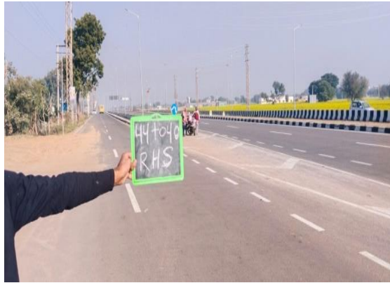
Fig 4.115: Service road at Ch 44+040 RHS
