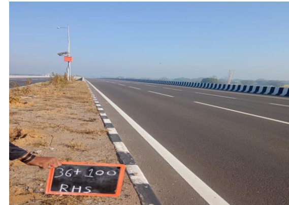
Fig 4.224: Camera with solar panel at Ch 36+100
