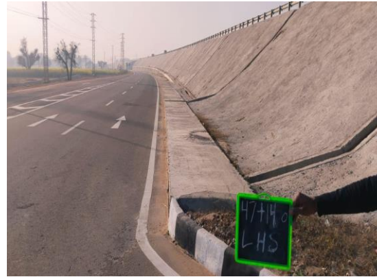
Fig 4.179: RCC Toe Drain at Ch 47+140 LHS
