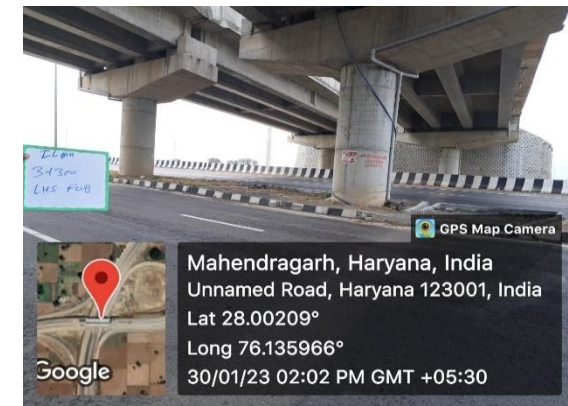
Fig 4.345: Flyover at Ch. 3+300 LHS
