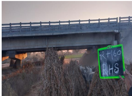
Fig 4.267: MNB at Ch. 42+160 RHS
