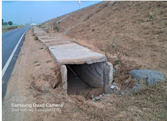
Fig 4.190: RCC Toe Drain at Ch 1+600 RHS
