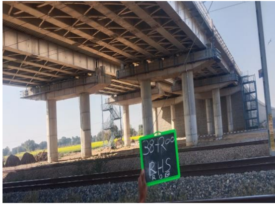
Fig 4.350: ROB at Ch 38+200 RHS
