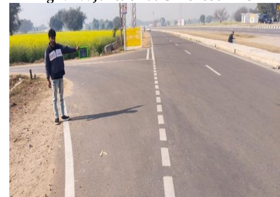
Fig 4.132: Junction at CH 52+900 LHS
