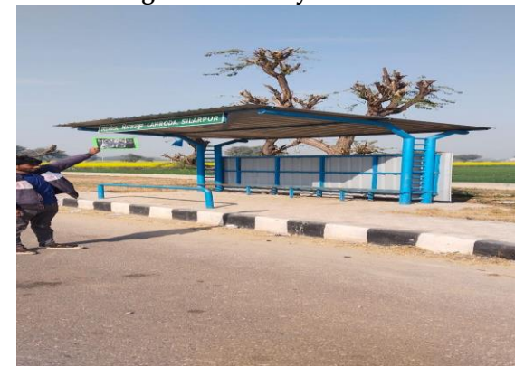
Fig 4.162: Busbay at 46+740 RHS
