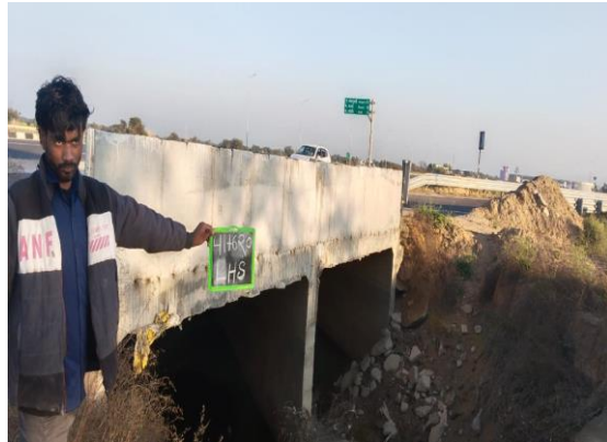
Fig 4.264: MNB at Ch.41+620 LHS
