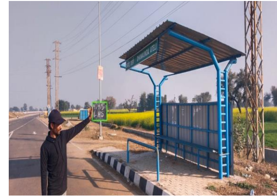
Fig 4.165: Busbay at 47+150 LHS
