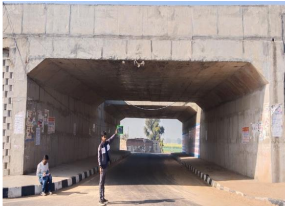
Fig 4.314: LVUP at Ch.30+250 RHS
