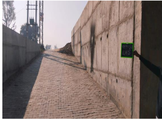
Fig 4.318: Subway at Ch. 46+580 LHS
