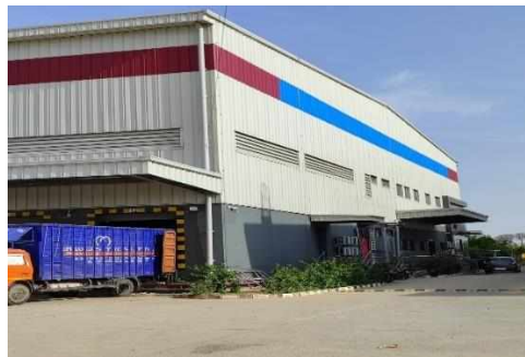
Rewari Road, NH-71, New NH 352, Chainage Rd, Gijarod – Jhajjar (Sr No 41)
