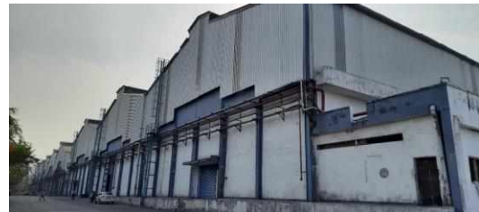
New Era Warehousing and Industrial complex, Lohop, /Vanivali, Patalganga, Rasayni, Raigad District (Sr No 38)
