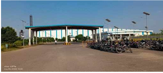
Sultanpur NDC, Industrial Plot No 1, Village: Dadri Toe, Jhajjar – Haryana (Sr 18)
