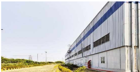
Building No. B-400, Indospace Sugar Industrial Park, Koodapakkam, Poonamallee, Tiruvallur (Sr No 47)
