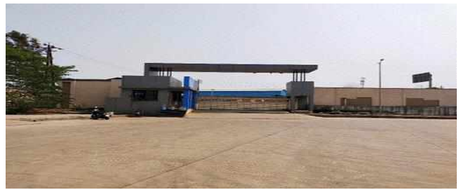
Saptshree Warehouse, Vahuli village Tel - Bhiwandi (Sr 3)
