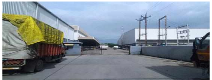
Sumar logistics and Industrial park, NH-8, Village Hariyala, District - Kheda (Sr 6)
