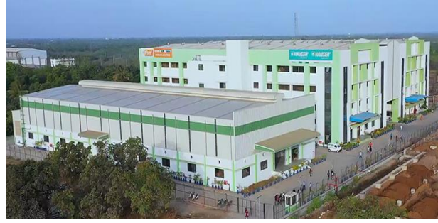
Valsad Building-II and Valsad Building-III
