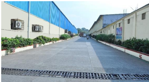
Sagar Complex, Ovali, Bhiwandi, Dist. Thane (Sr No 39)
