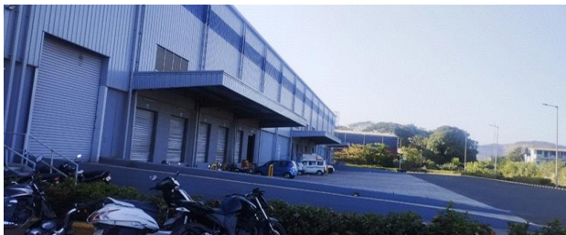
Building No B200, Shed 200, Indran Logi Indospace Industrial & Logistics, Ajivali, Khalapur Raigad - Khopoli (Sr No 21)
