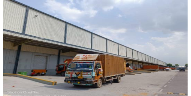
Embassy Industrial Park, 122506 Farukhnagar – Haryana (Sr No 28)
