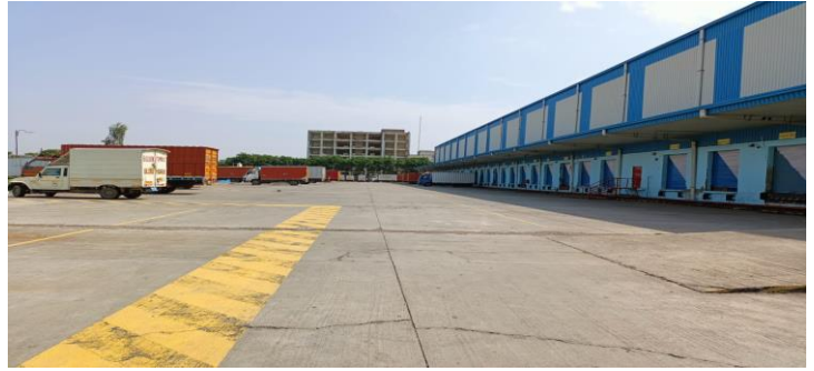
Kharasa No 1243/1218 Khewat No 295/294/289 Khatoni No 364/365 & Khewat 359/363 Hadbast No 346, Shambhu Kalan, Rajpura, Punjab (Sr No 62)
