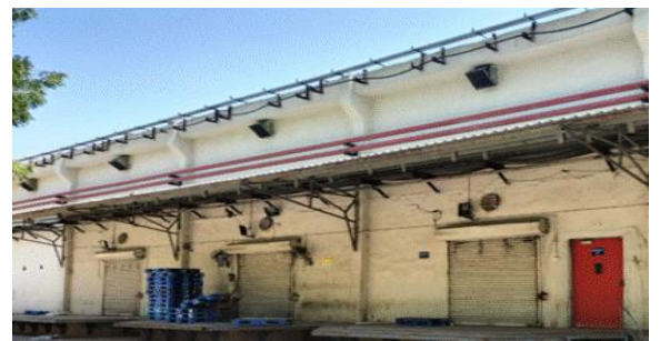
Gate No 5,GIDC Naroda - Ahmedabad (Sr 17)
