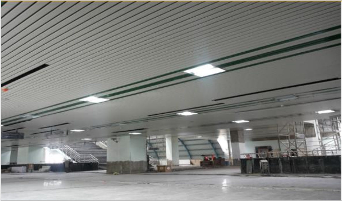
(b) Metal roofing and cladding systems
