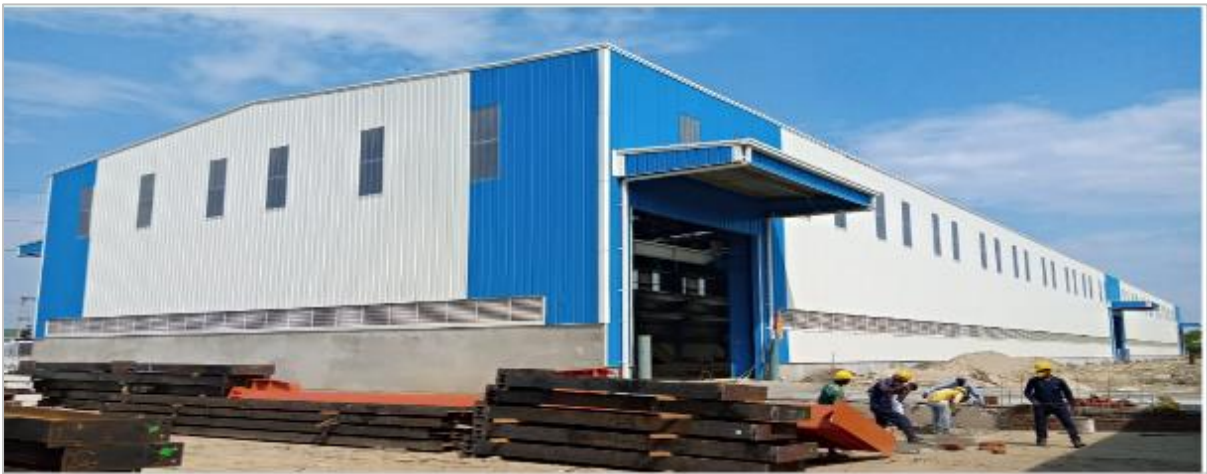
Tamil Nadu Manufacturing Facility I
